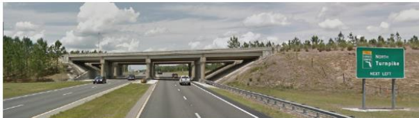
US 27 at Florida's Turnpike/SR 91 (Bridge #110006 and 110073)
