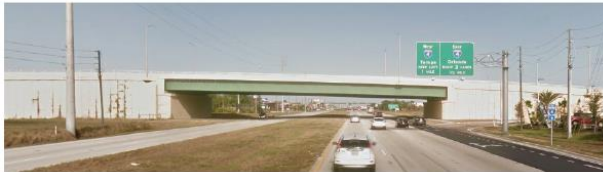
US 27 at Ernie Caldwell Boulevard (Bridge #164536)
