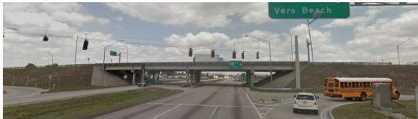
US 27 at SR 60 (Bridge #160134 and 160018)
